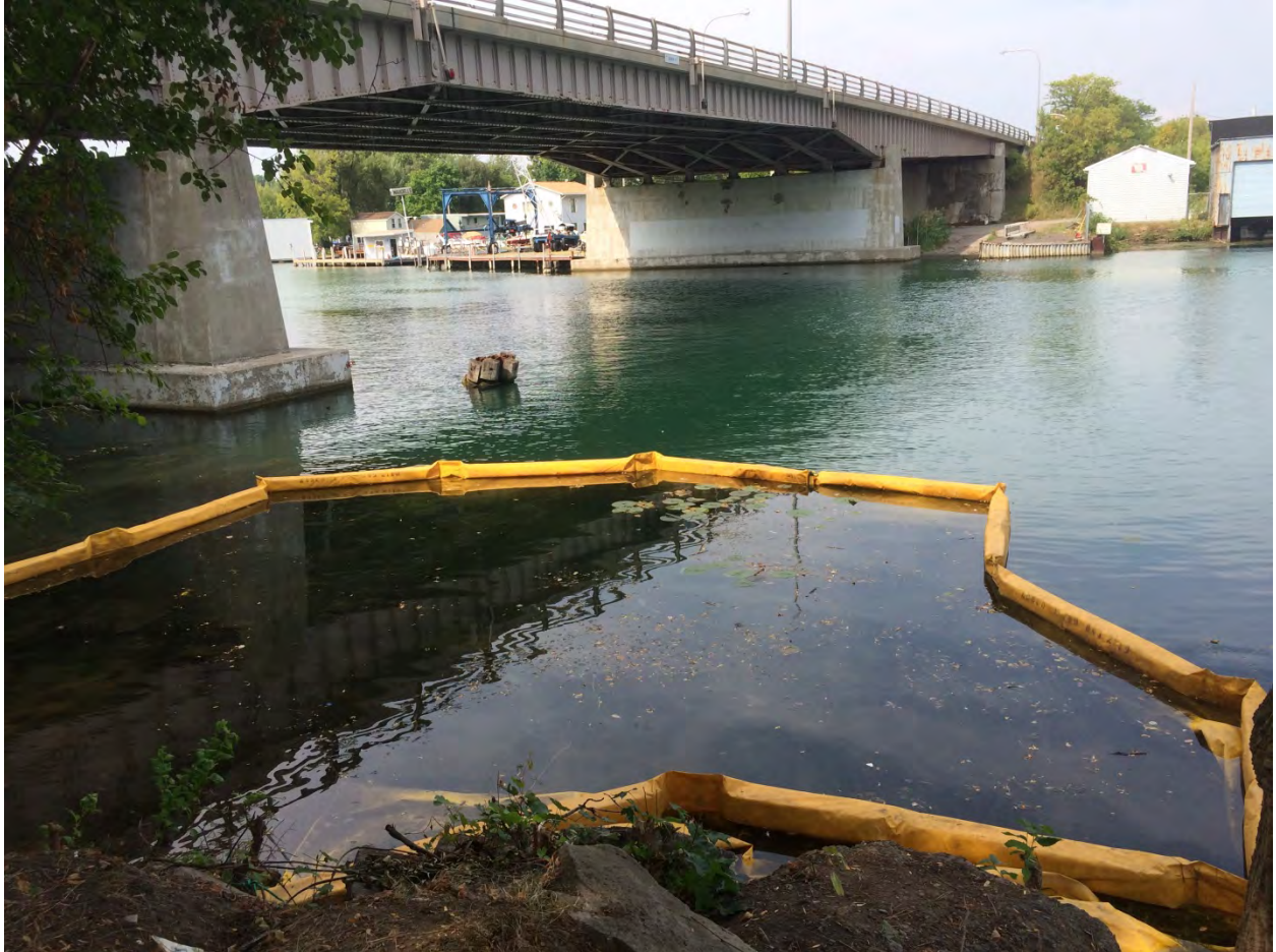
Photo A-6 Spot treatment area.
